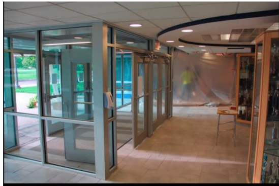
Secure Entrance being built at the high school
